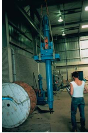
Flood gate regulation
