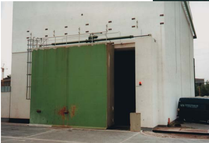
Gate actuator Force: 10 t, Stroke: 7000 mm
